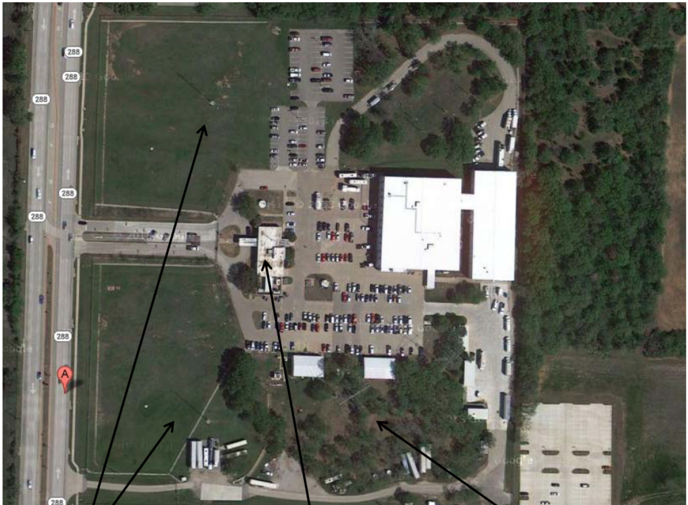
Aerial view of FEMA, Federal Regional Center (FRC) site at 800 N Loop 288, Denton, Texas
